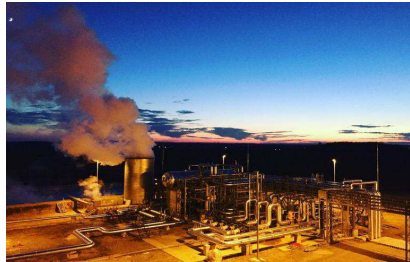
Velika Ciglana geothermal plant; Source: Turboden
