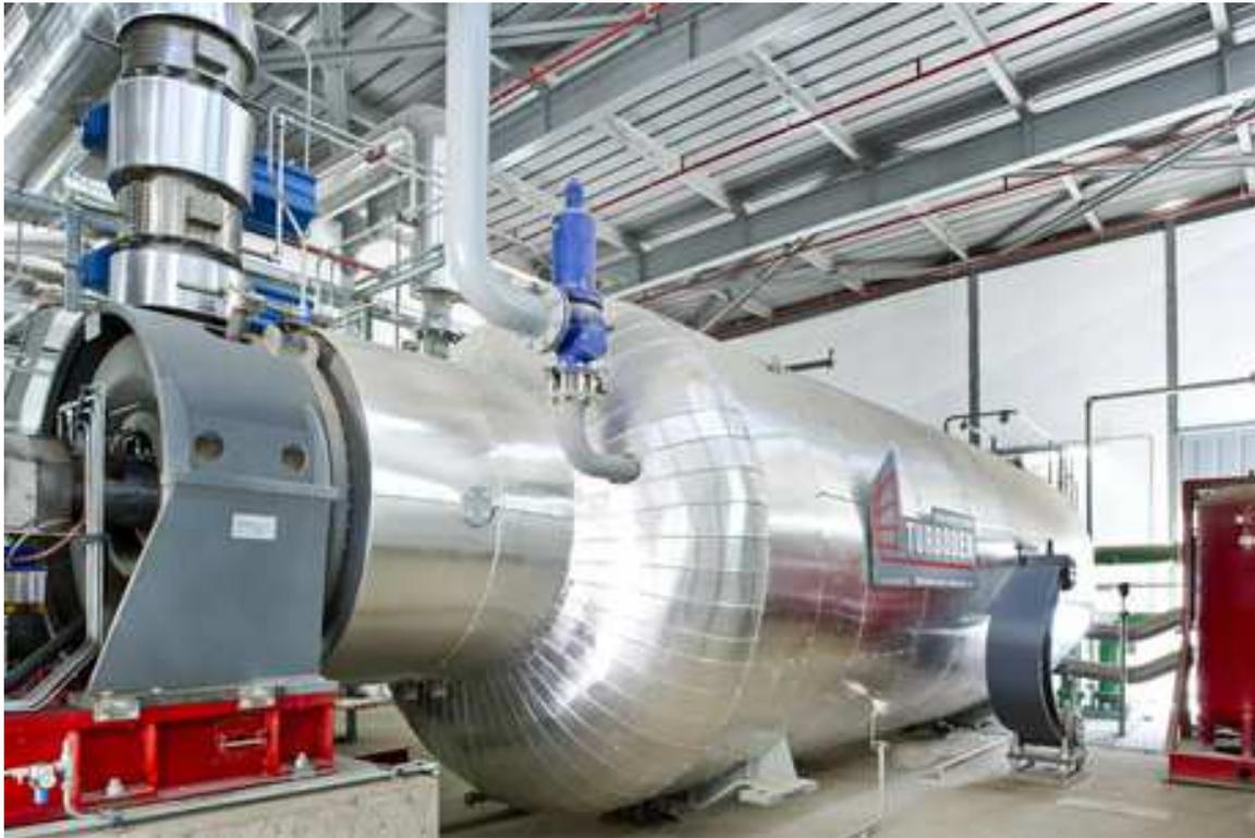
A Western Australian oat miller is using the Organic Rankine Cycle (ORC) turbogenerator system from Italian company Turboden to generate clean electricity using oat husks as fuel to power its Wagin facility.
