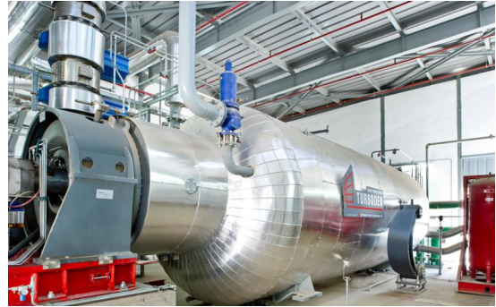
ORC turbogenerator by Turboden.
