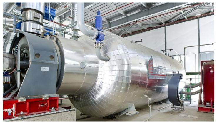
The ORC unit is a system based on a closed-loop thermodynamic cycle for the generation of electric and thermal power, especially suitable for distributed generation (photo: Turboden)
