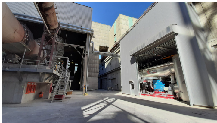
Turboden's 1.3 MW ORC module at Holcim Eclépens facility, in Switzerland. The ORC is fed by superheated water, which is also used to supply the district heating network of the town near the plant.
