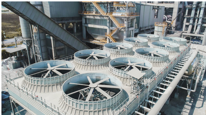
Turboden's ORC power plant for Sönmez Çimento in Turkey. In operation since 2020, the unit generates 7.3 MW by exploiting the pre-heater exhaust gases and the hot air from the clinker cooler.
