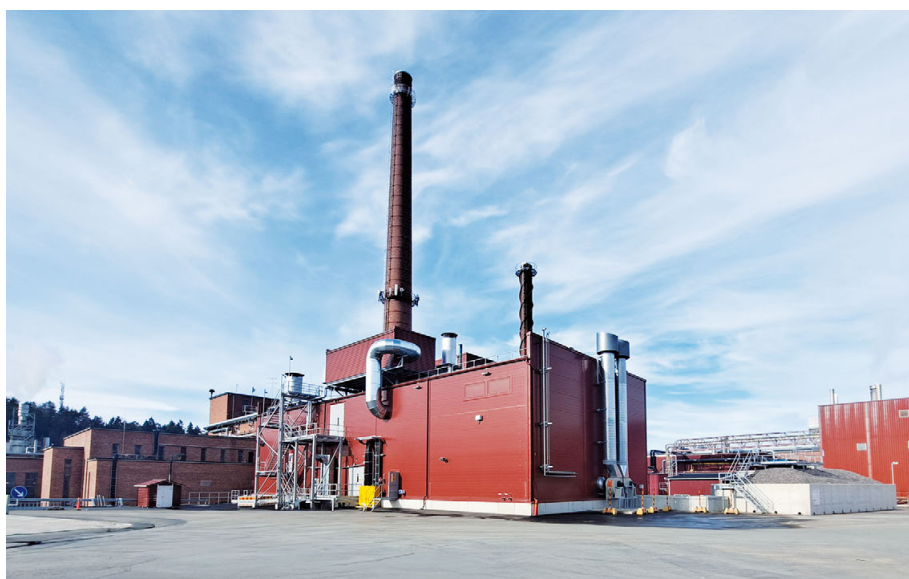
Fig. 1. External view of the delfort heat pump.
